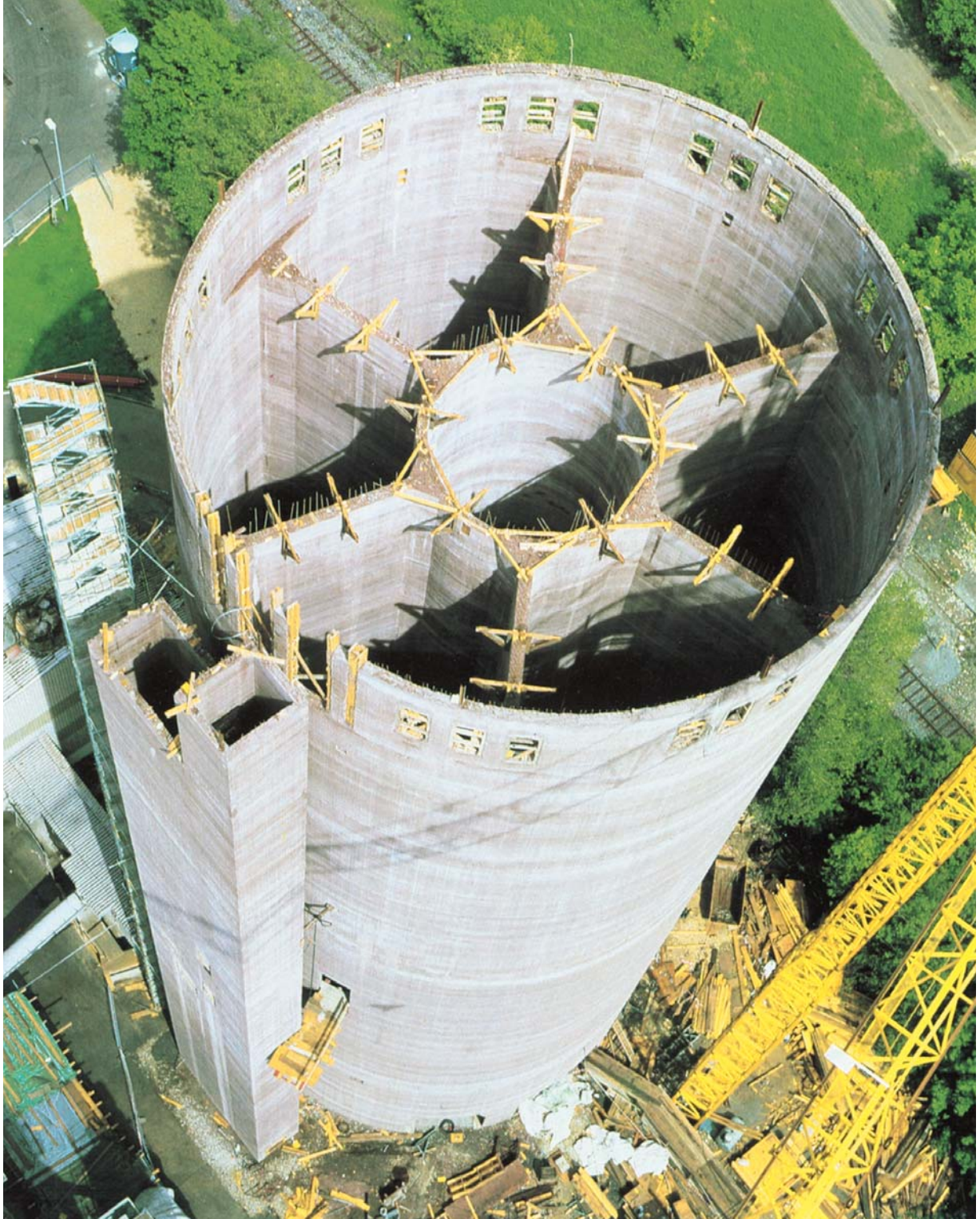
Multi-compartment cone silo
