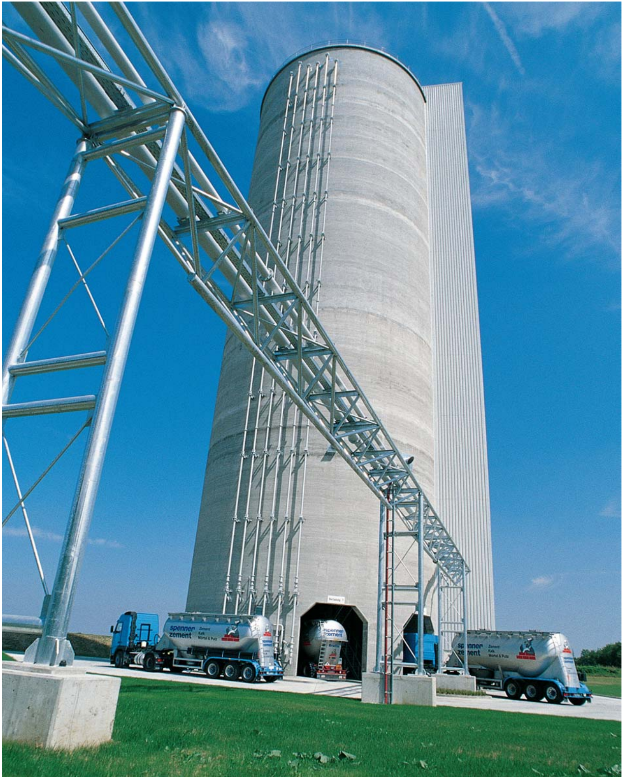
SPENNER ZEMENT Multi-compartment silo, Germany
