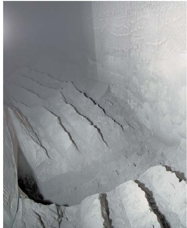
The emptying rate of the silo is more than 99 %
