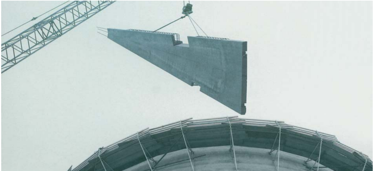
Lifting of cone segments
