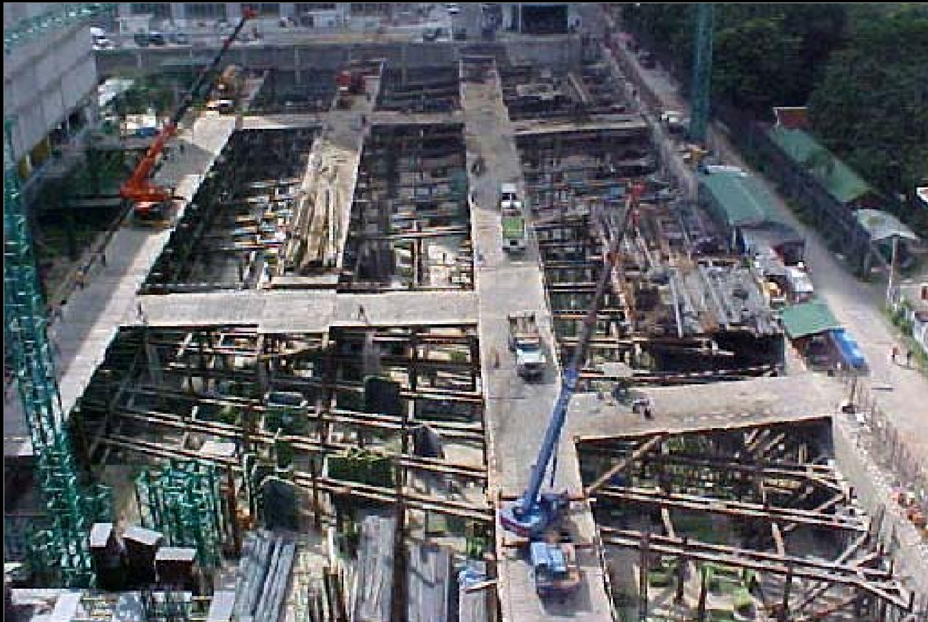
SHEET PILE W/ BRACING
