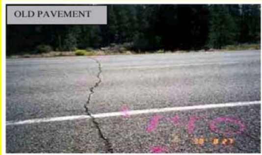
Crack 140 (transverse) in September 1998 before overlay
