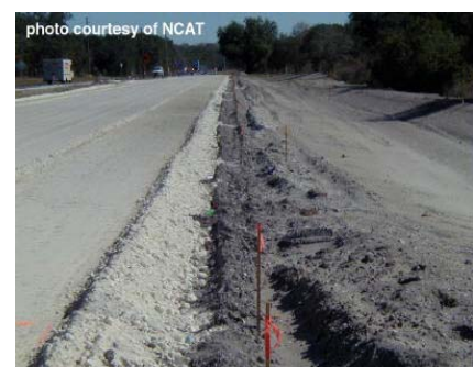
Figure 3: Limerock Base Course Undergoing Final Grading
