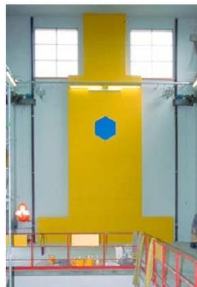
New reinforced concrete structural wall from the inside of the east facade of the assembly shop.
