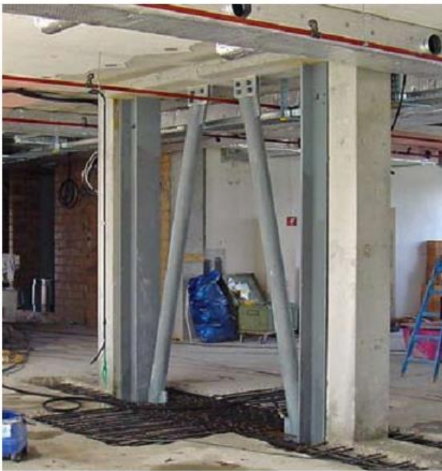
New eccentric steel framework constructed between two existing reinforced concrete columns.
