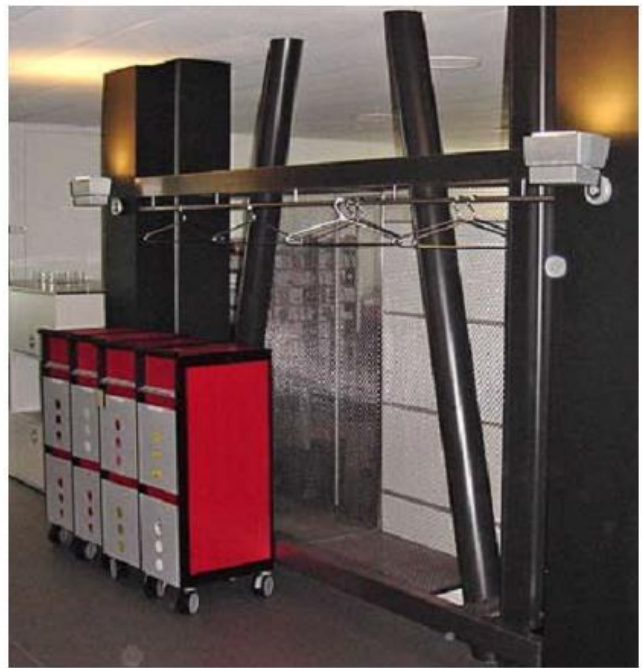
New eccentric steel framework with a column disguise.
