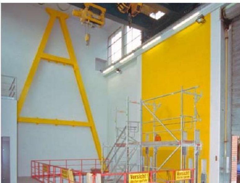
New A-shaped steel frame on the west facade and new reinforced concrete structural wall on the north facade of the assembly shop.
