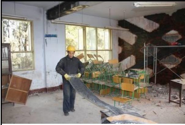
Strengthening of walls, beams and columns
