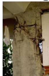
Shear failure of column
