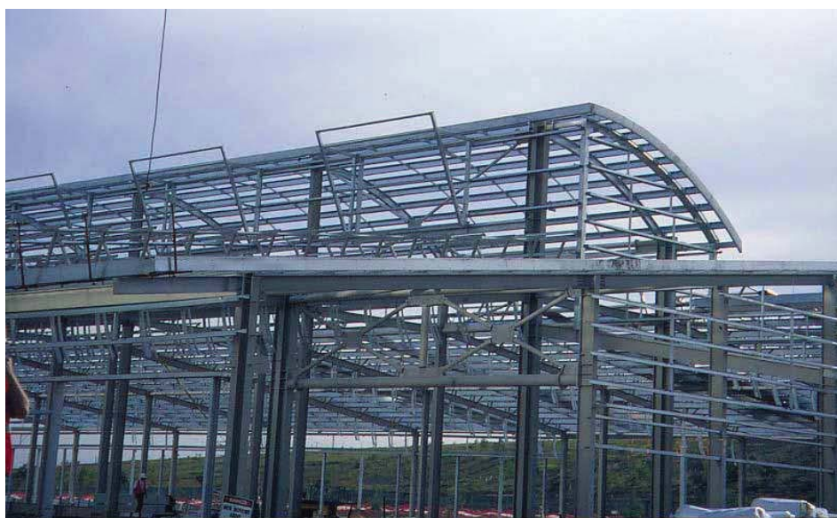
Roof and Walls
