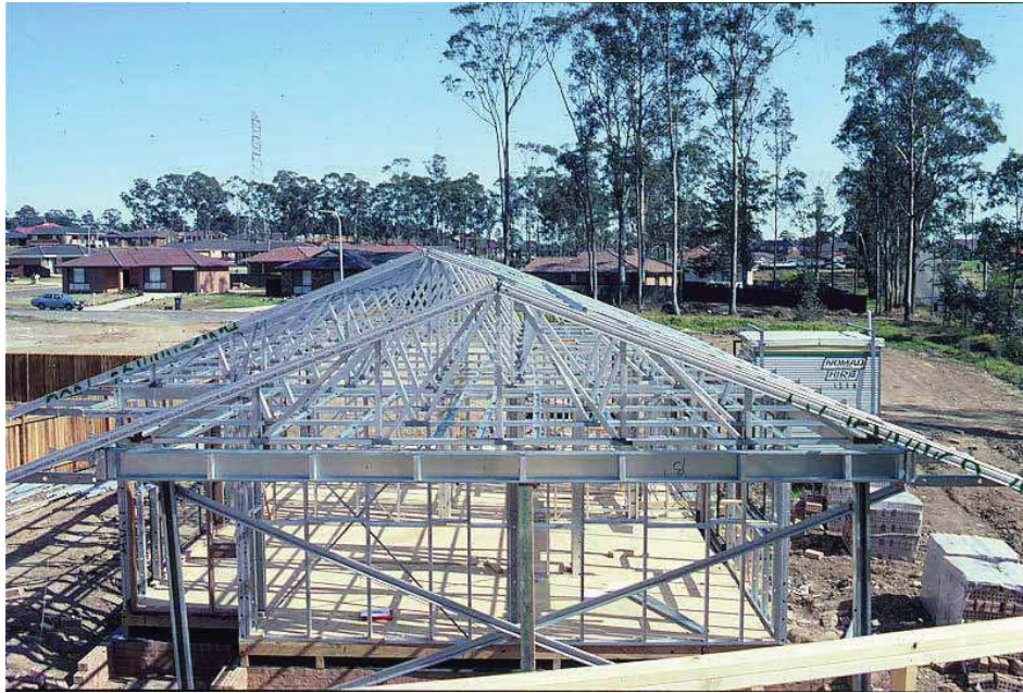
Steel Framed House
