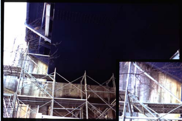
Railway bridge, Sannomiya, Kobe, 1995 Photo from EASY
