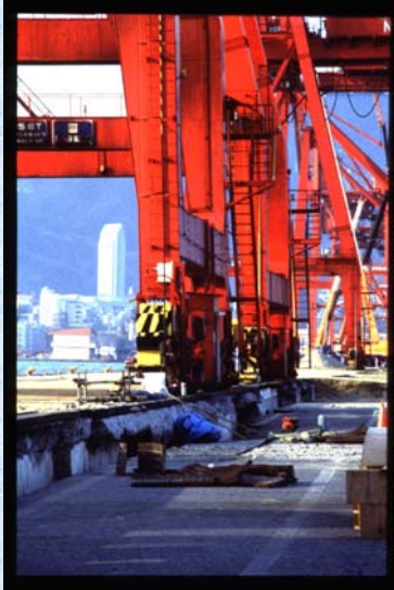
Large settlements of ground near crane girders on piles. Kobe 1995 Photo from EASY
