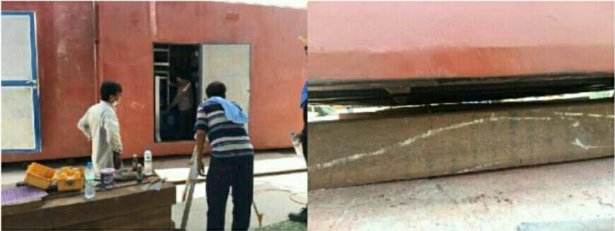
Structure deflect measuring by Level measuring device
