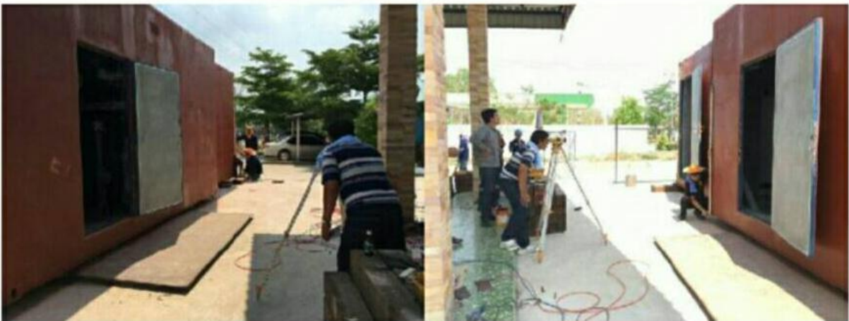
Structure deflect measuring by Level measuring device
