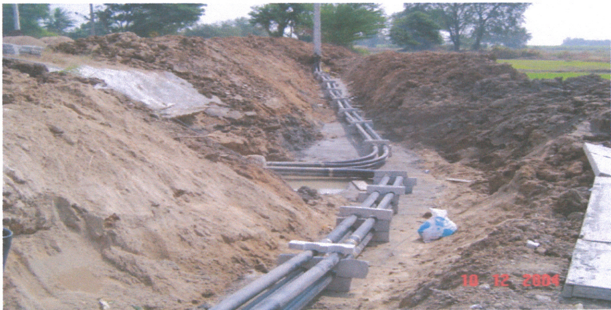
HDPE PIPE WITH DUCT BANK
