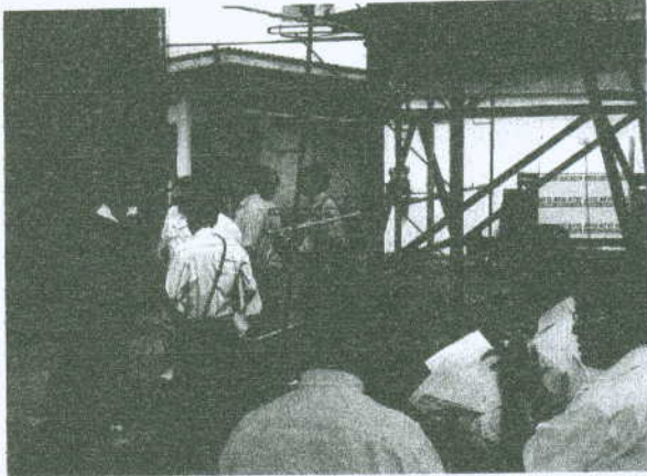
Photo 8. Inspection of mock-up sample
