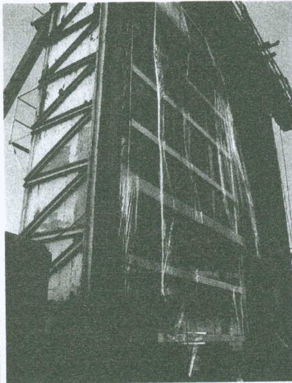
Photo 10. Polythene sheet for Air Infiltration test
