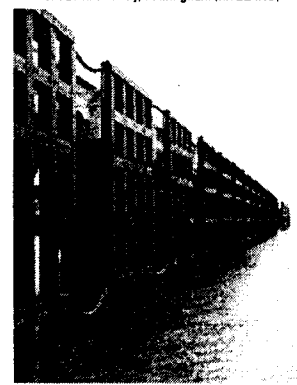
▼ West Lead-In Jetty, Immingham (ENGLAND)
