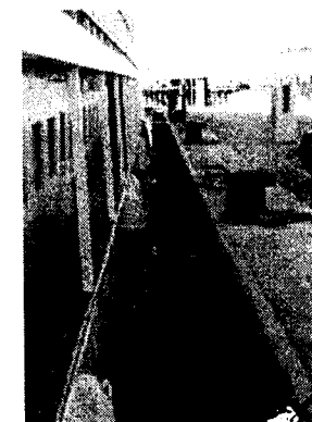
▲ Passenger Quay, Mukran (GERMANY)
